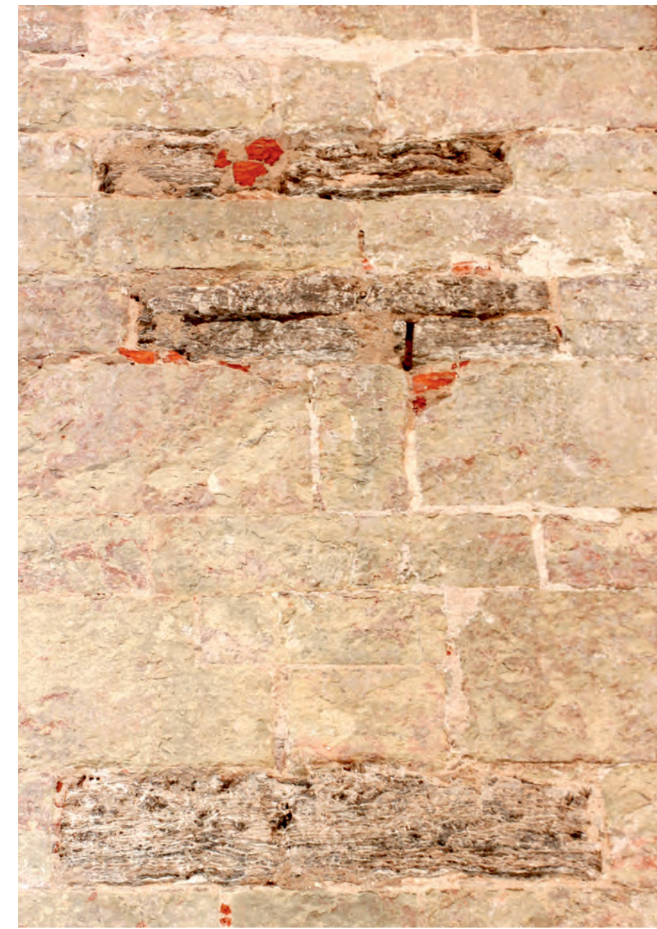
1., 2. Gypsum stone blocks in the Northern wall pilaster of Riga Cathedral, XIII c.
