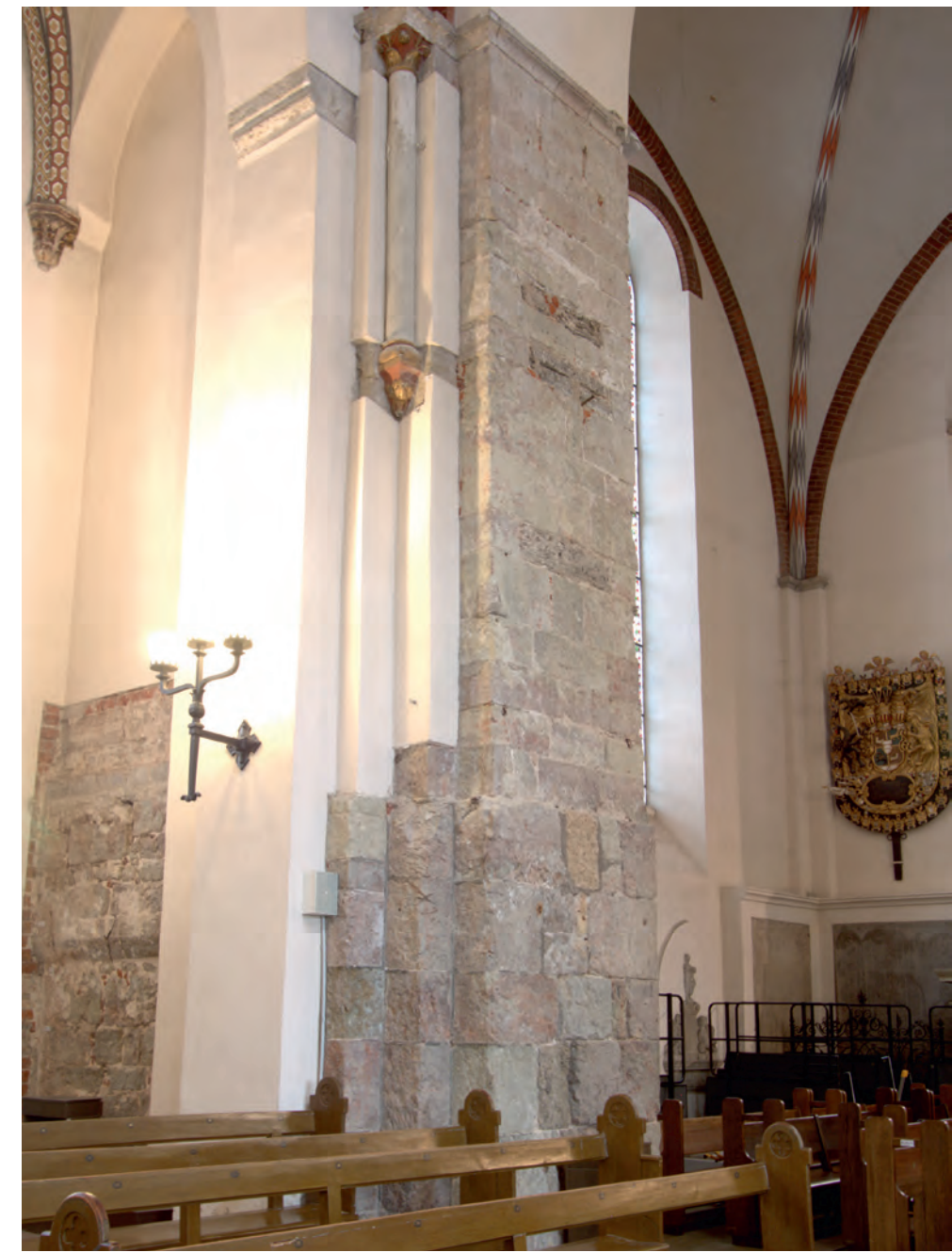
1., 2. Gypsum stone blocks in the Northern wall pilaster of Riga Cathedral, XIII c.
